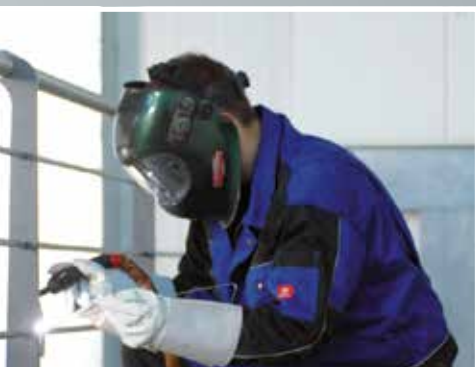
2. Steel / stainless welding in DC
